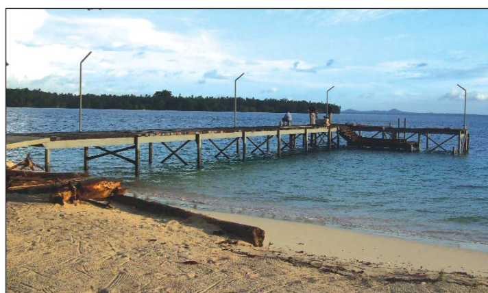
• The completed fisheries jetty on much talked-about Nango Island Mari culture Facility, Kavieng, NIP
