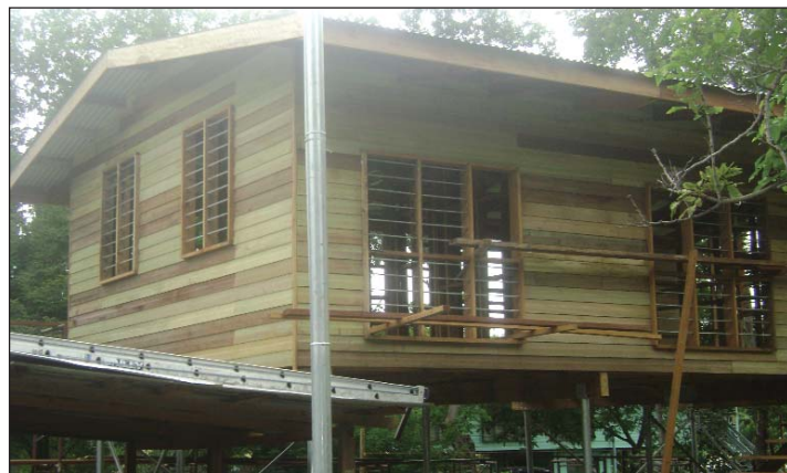
• This is one of the three bed room houses under construction at Kanudi estate in Port Moresby. (Picture by Steven Poning)
