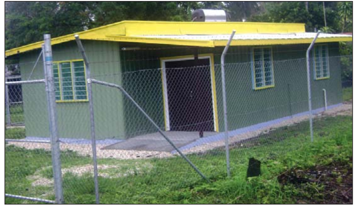
• The refurbished Finschhafen District Fisheries Office.
